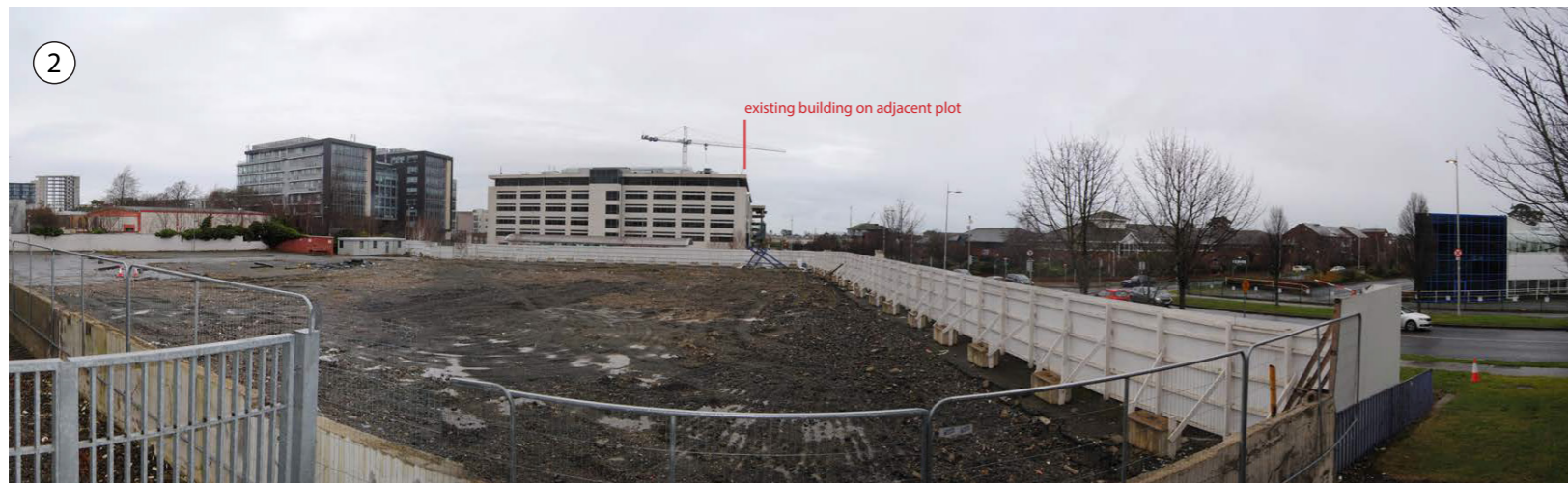
Current internal view looking north with former building demolished
