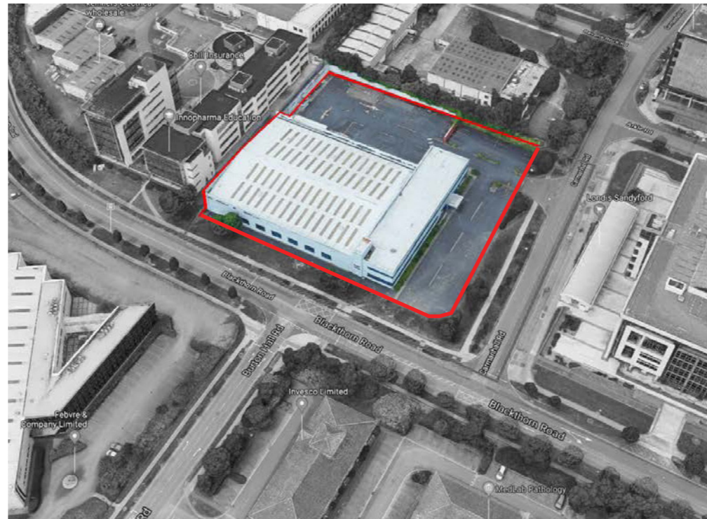
Aerial view of site with former commercial building looking west
