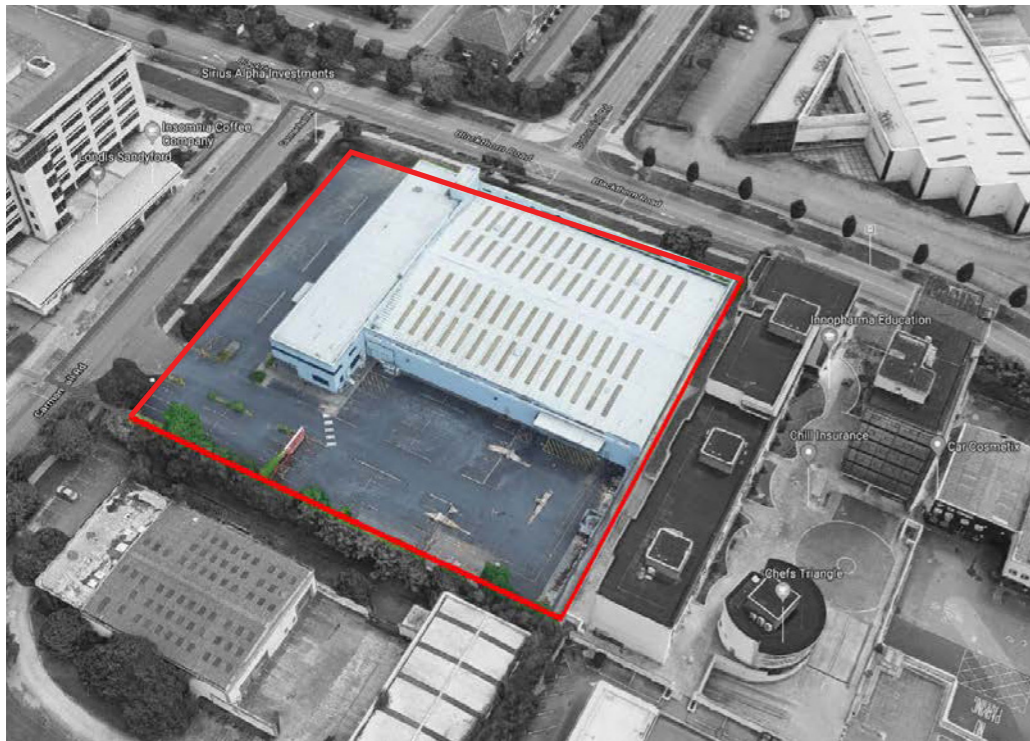
Aerial view of site with former commercial building looking east
