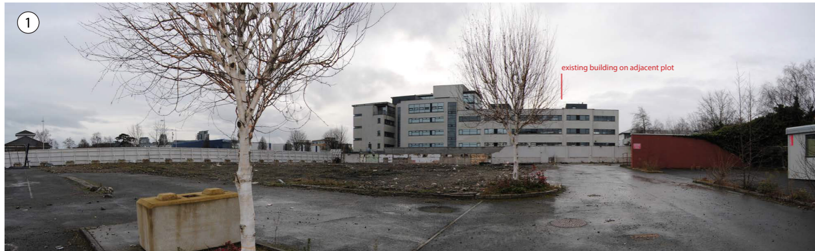
Current internal view looking south with building former demolished
