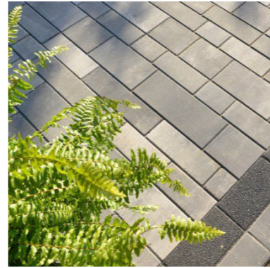
HIGH QUALITY PAVING
